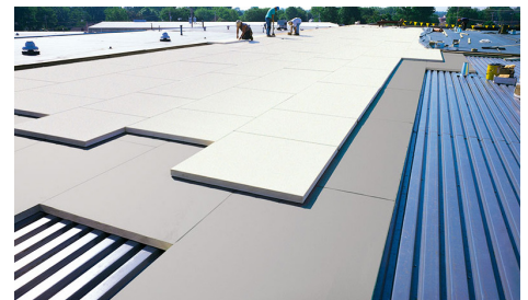
Polyiso roof insulation on a commercial building.
